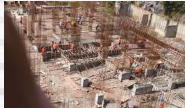
PHOENIX MALL - RCC WORKS
