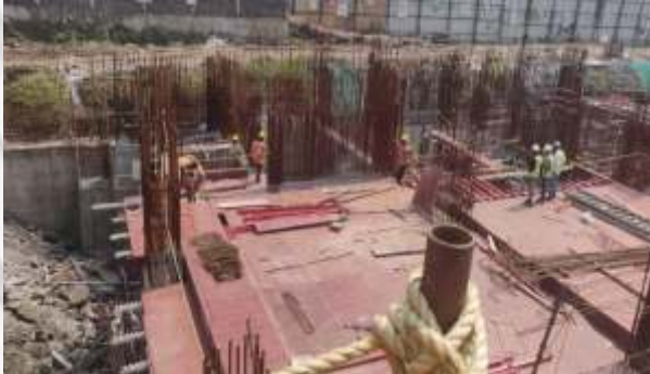
PHINIX MALL-RCC WORKS (SHUTTERING STEEL & CONCRETE)
