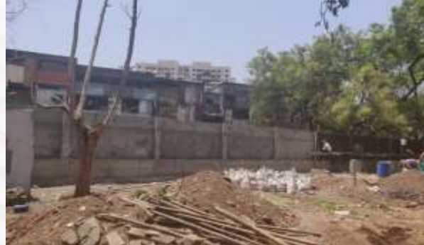
SUGANDHA LAWS - RCC BOUNDARY WALL
