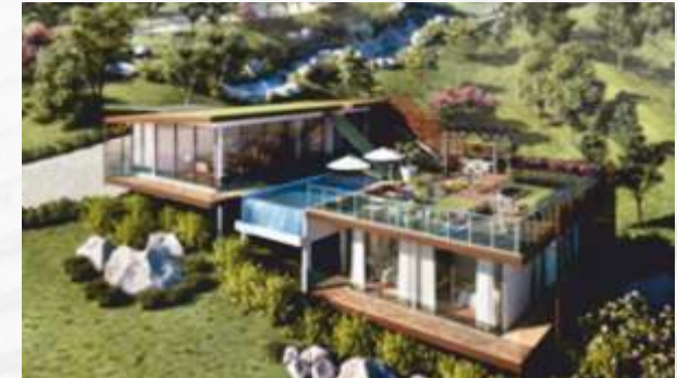
ALTERRA – AT PAWNA DAM, LONAVALA
