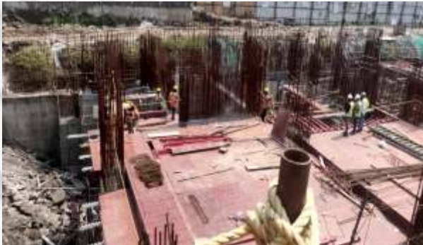
PHOENIX MALL - RCC WORKS
