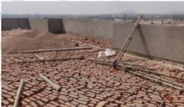
WATER PROOF WORKS @VT PARLESHA-KHARADI
